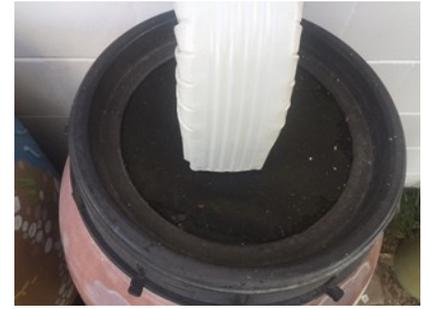
A RAIN BARREL WITH A TIGHTLY SEALED LID AND SCREEN .
