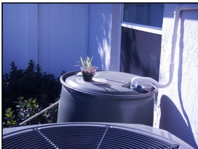
A RAIN BARREL COLLECTS CONDENSATE FROM AN AIR CONDITIONER UNIT.
